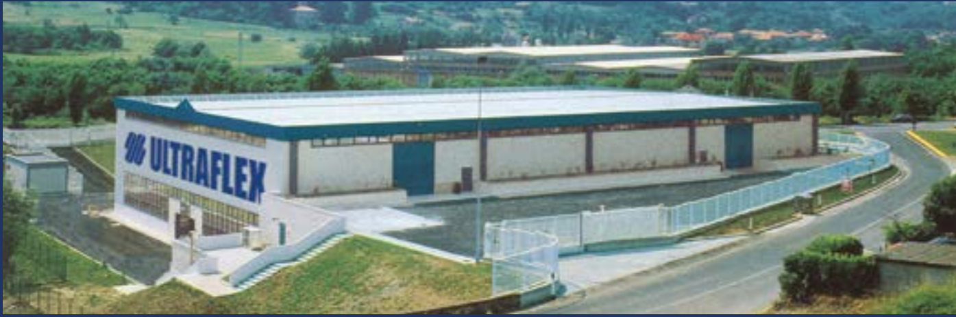
ULTRAFLEX Casella factory
