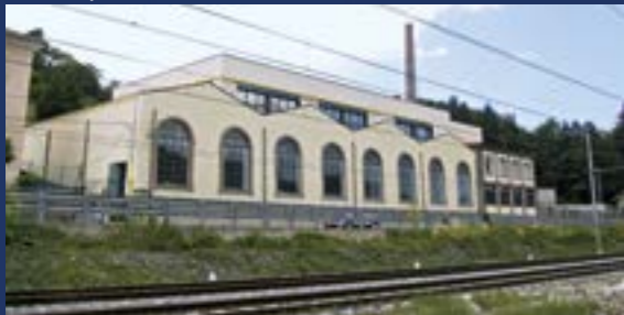
UCS - Ultraflex Control System Borgo Fornari factory
