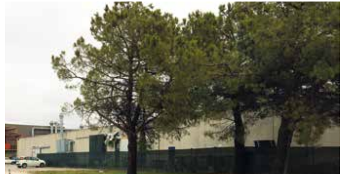
UFLEX - Factory in Tregnago
