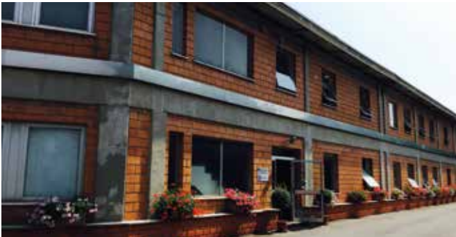
UFLEX & ULTRAFLEX - Headquarter in Busalla
