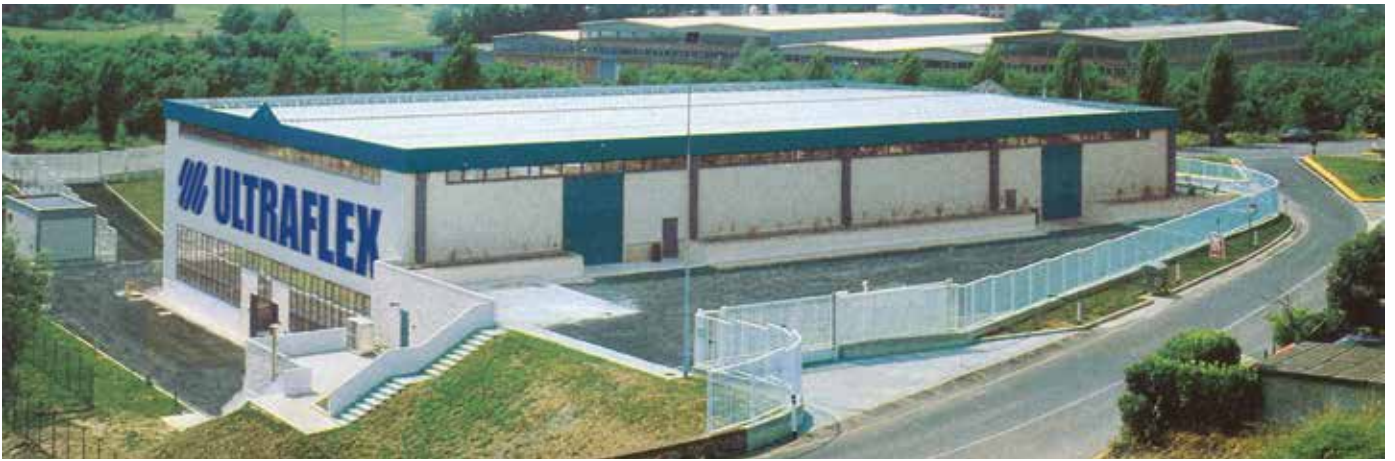
ULTRAFLEX - Factory in Casella
